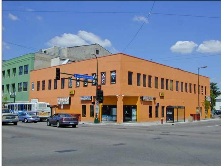
Panaderia San Miguel, formerly the Butler Drug store, at 1518 East Lake Street. KFAI relocated its studios to this building in 1986.
